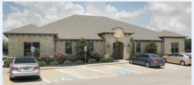
ASA's National Headquarters North Richland Hills, Texas
